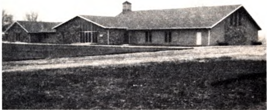
The new facilities of Bicknell, Ind., First Church were dedicated Sept. 9, 1979, with Dr. B. G. Wiggs, district superintendent, bringing the dedicatory message. The new sanctuary, educational unit, and fellowship center is 10,000 sq. ft. and was erected for one-half its value of $325,000. The building is wood frame with brick/stone veneer. The sanctuary, with sloping floor, laminated arches, and spring cushioned pews, has a seating capacity of 400. Joseph F. Webb was the consulting engineer and Rev. Sylvanus Carter was the builder. Men of the local church accepted responsibility of particular phases of the construction. Rev. Bill L. Reed has served as pastor since 1975.
