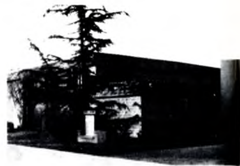
The new sanctuary for the Orange, Calif., church was dedicated November 30. Dr. Nicholas Hull brought the dedication message, and Rev. Robert Scott, district superintendent, prayed the prayer of dedication. The sanctuary has 5,500 square feet, with seating capacity of 360. Total cost for the sanctuary is about $175,000. This new addition brings the property value of the church to nearly $350,000. The church is completing 18 years of ministry in Orange. Rev. Richard Graley has been the pastor for the past 10 years.
