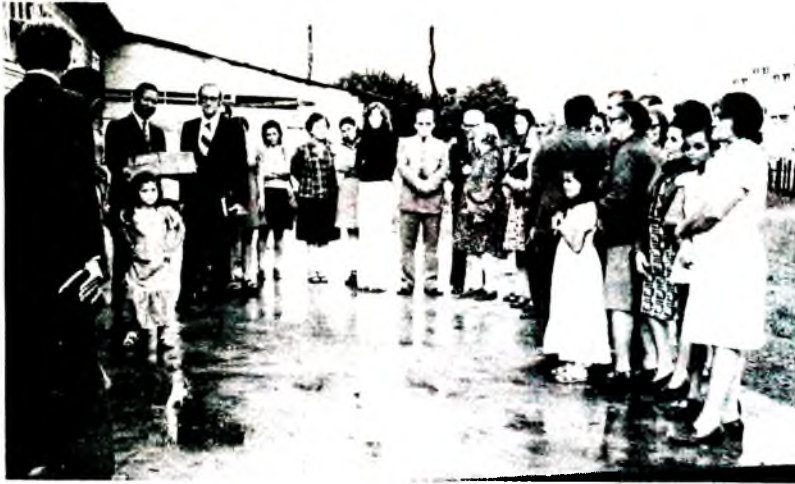
The contractor holds a special box to go in the cornerstone of the new Brasilia Church of the Nazarene.
