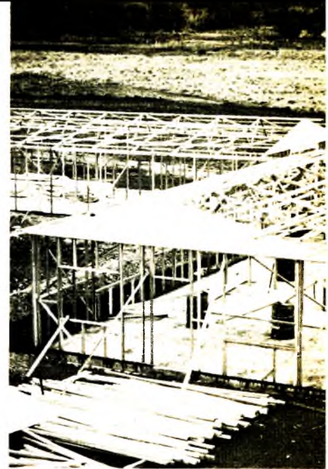
Rough construction under way for kitchen and storage area.
