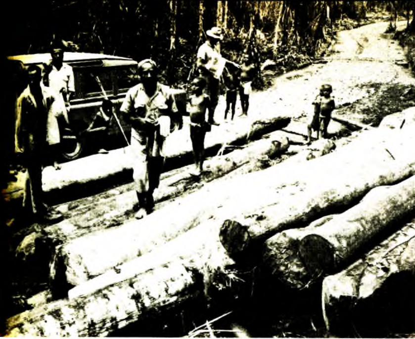
Logging crew begin their long tour back down the road they helped construct with timber for the hospital.
