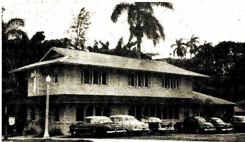
Our church and parsonage at Ancon, Panama Canal Zone, Rev. Elmer O. Nelson, pastor. The building has recently been enlarged, with the expense paid jointly by the Department of Home Missions, the local congregation, and an interested layman in California. The lower floor serves as sanctuary and for Sunday school. The pastor's living quarters are on the second floor.
